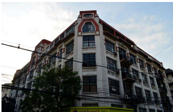
Present Day First United Building. Photo source: shaharaine.wordpress.com
